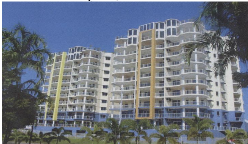
SYNERGY SQUARE, TWIN TOWERS
